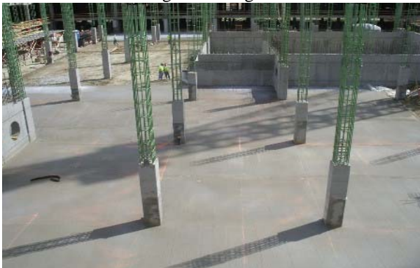
32,000 square feet of concrete placed April 24-25, 2009
