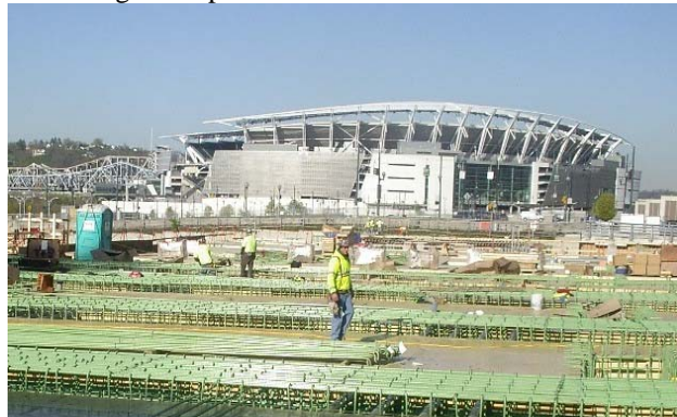
Freedom Way East rebar installation on elevated decking
