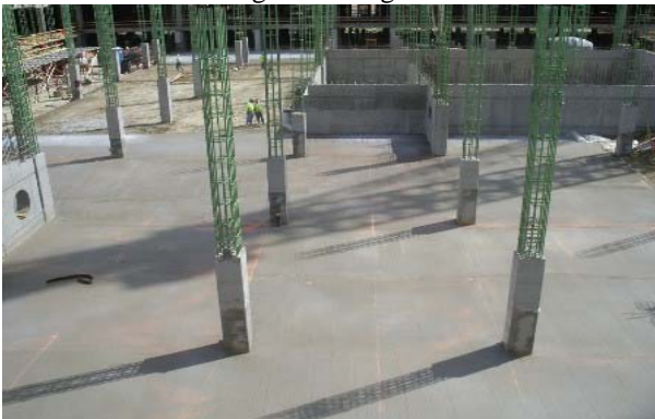
32,000 square feet of concrete placed April 24-25, 2009
