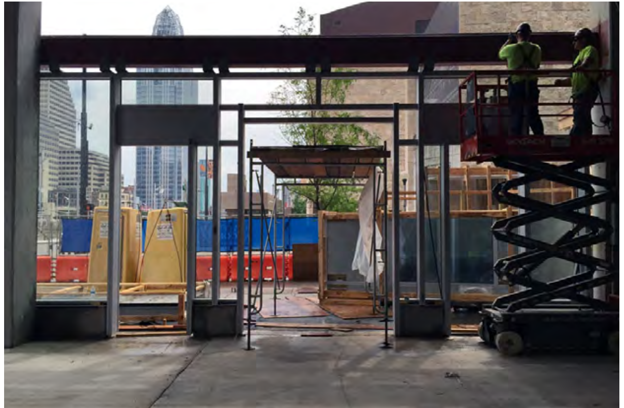
Glass is installed in the GE Building lobby.
