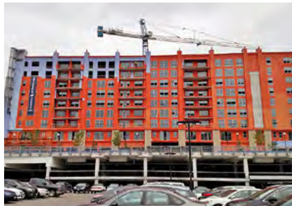
Apartment structure exterior skin cladding installation is underway.
