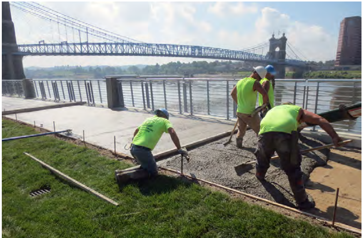
Workers smooth the fresh concrete along the Ohio River Walk.
