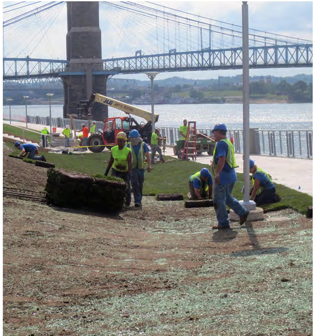
Workers install sod along the Ohio River Walk.
