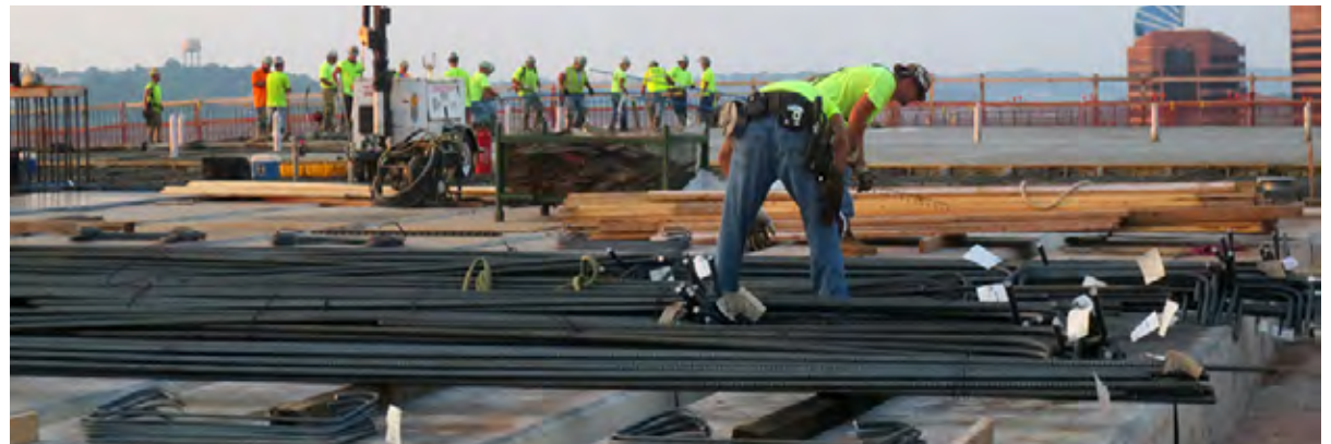
GE Building top deck construction ('all hands on deck').
