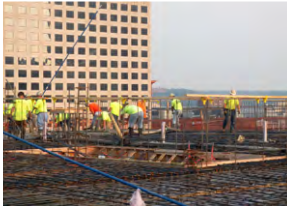
Workers prepare for the final concrete pour on the GE Building.
