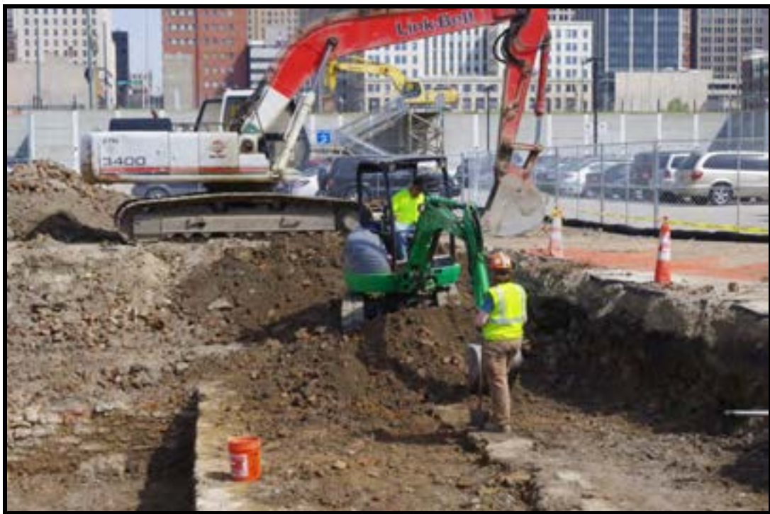
Plate 1. Excavation block showing large trackhoe and mini excavator, facing north.
