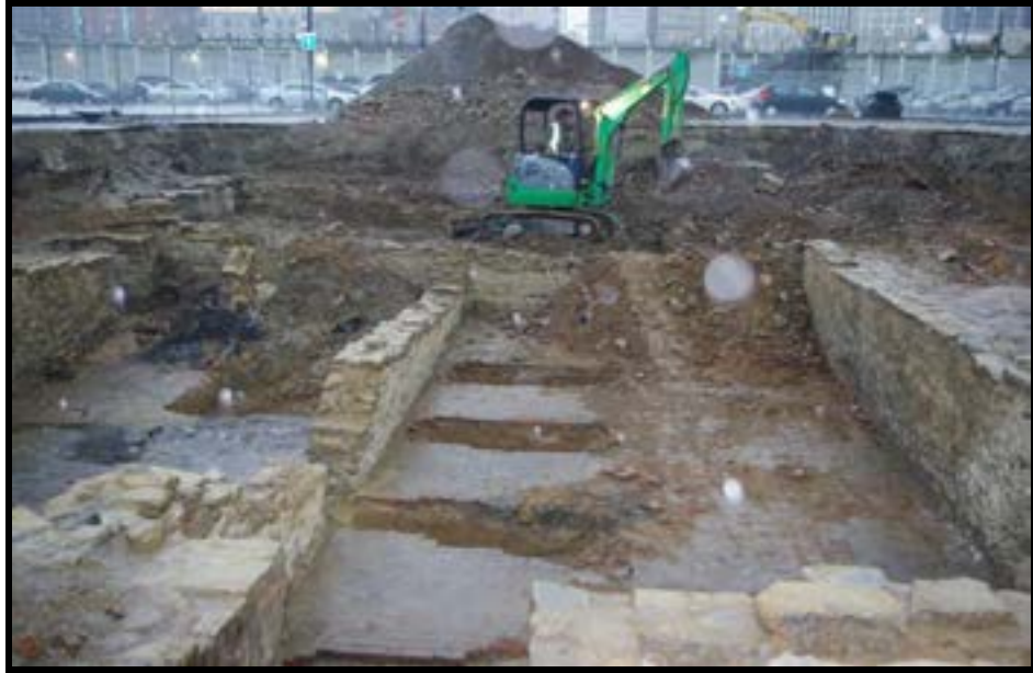
Plate 7. Exploratory trenches excavated beneath the basements of 116 and 118 Water Street, facing north.
