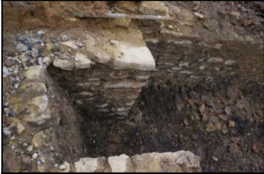
Plate 5. Top view of the opening uncovered in the northwest corner of 118 Water Street, facing down.
