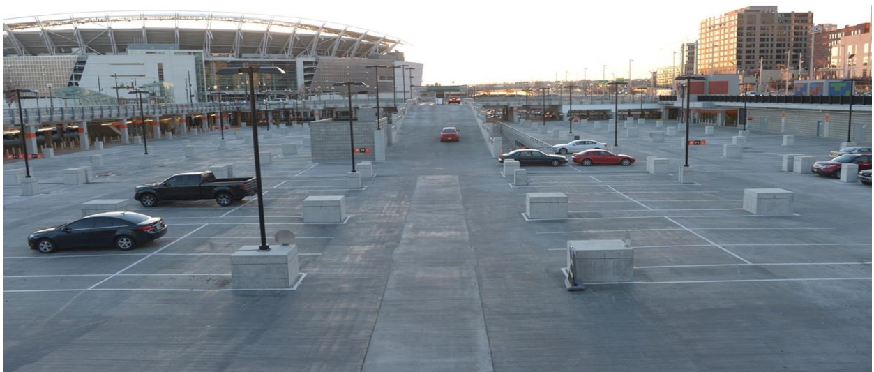
Lot 24 Looking West Towards Paycor Stadium
