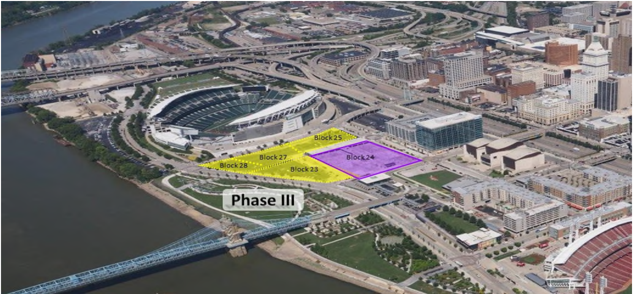
Figure 17 - Phase III of The Banks Intermodal Transit Facility; Federal Funding will be applied to the construction of Lot 25.
