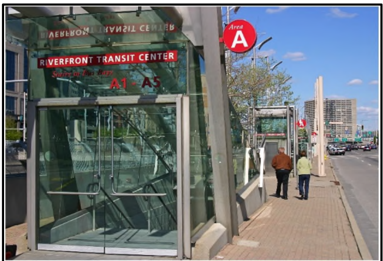
Figure 12 - Second Street entrances to the Riverfront Transit Center
