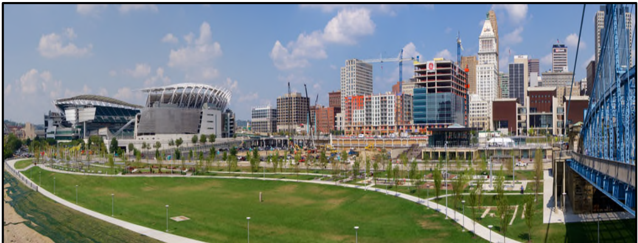
Figure 32 - The Banks Mixed Use Development
