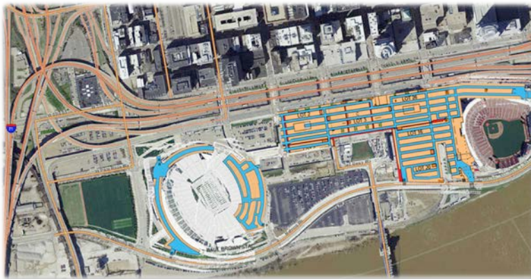
COMPLETED PHASES OF BANKS INTERMODAL TRANSIT FACILITY - 2012
