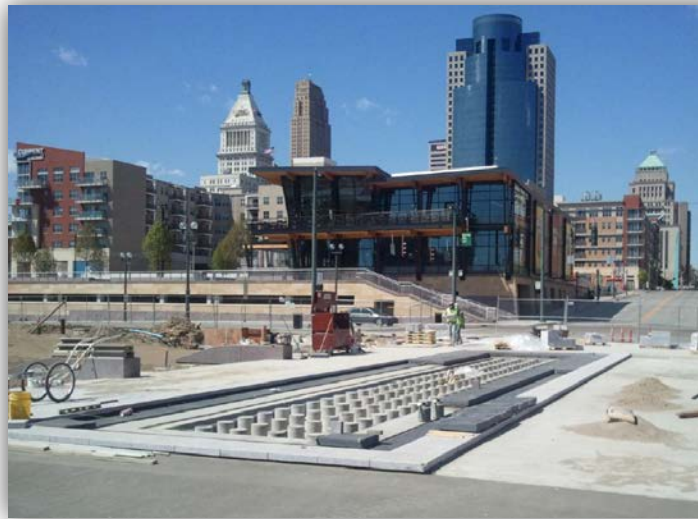
MOERLEIN LAGER HOUSE AND WALNUT STREET FOUNTAIN AT THE SMALE RIVERFRONT PARK – UNDER CONSTRUCTION
