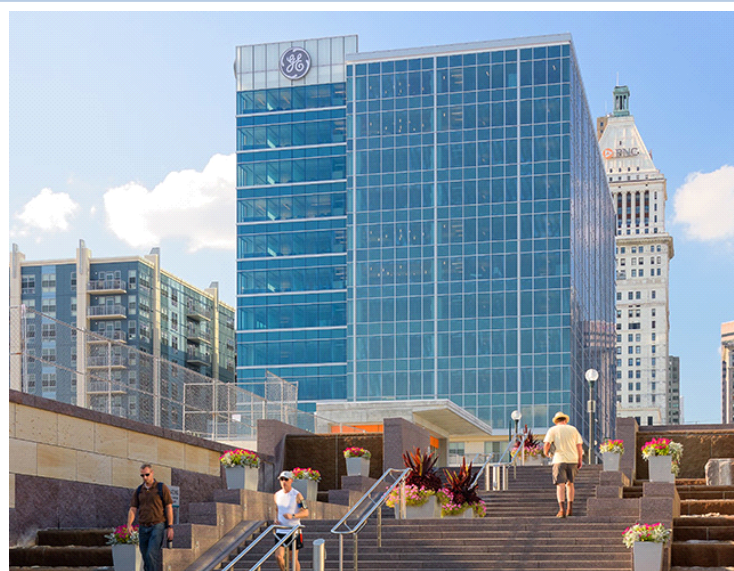
GENERAL ELECTRIC U.S. GLOBAL OPERATIONS CENTER @THE BANKS
