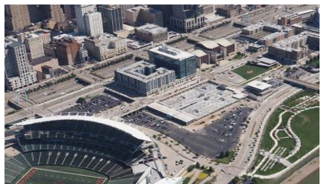
PHASE III CENTRAL RIVERFRONT GARAGE (WEST) SEPTEMBER 2017
