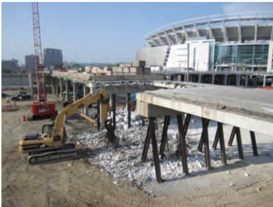
Photo #8 – Bid Package #11: Demolition of the Race Street Bridge Temporary Structure.
