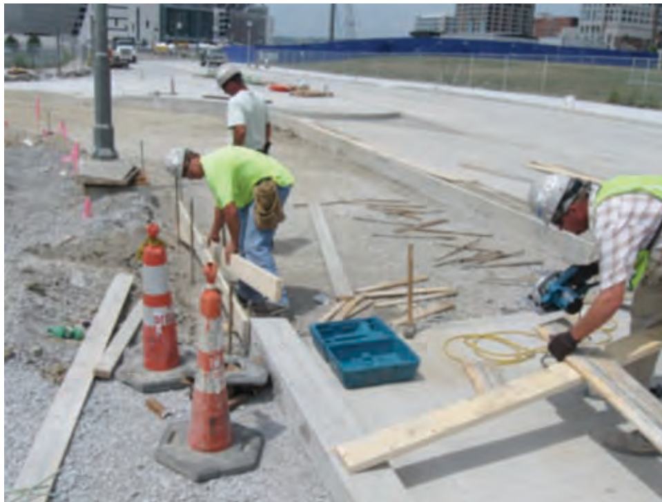
Photo #2 – Bid Package #9: Forming for pavement at Theodore M. Berry Way.
