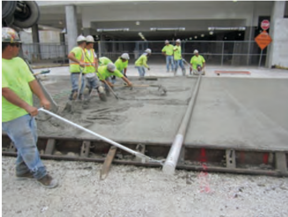
Photo #1 – Bid Package #9: Mehring Way pavement installation at Phase 1 Garage Entrance.
