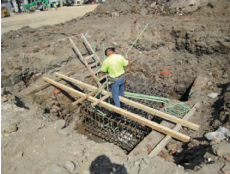
Photo #7 – Bid Package #11: Re-steel placement for pile cap installation.
