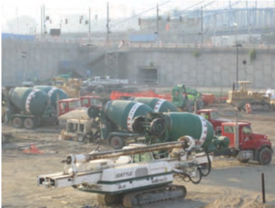
Photo #5 – Bid Package #9: Grout trucks lining up for pile installation.
