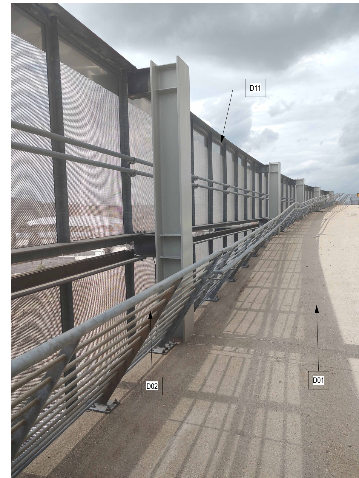
SECTOR 9 - LEVEL 700 RAMP
