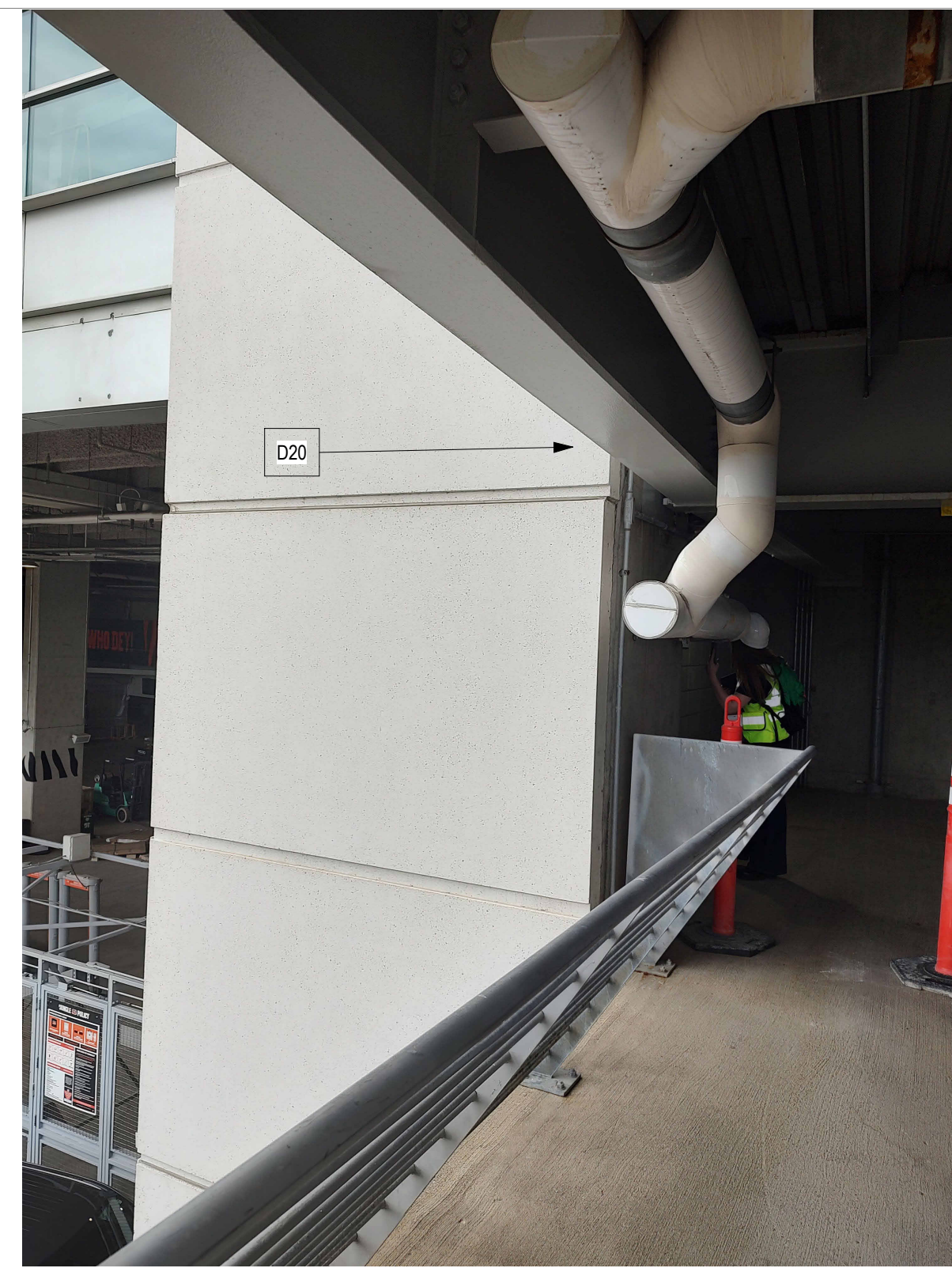
SECTOR 9 - LEVEL 350 NORTH LANDING
