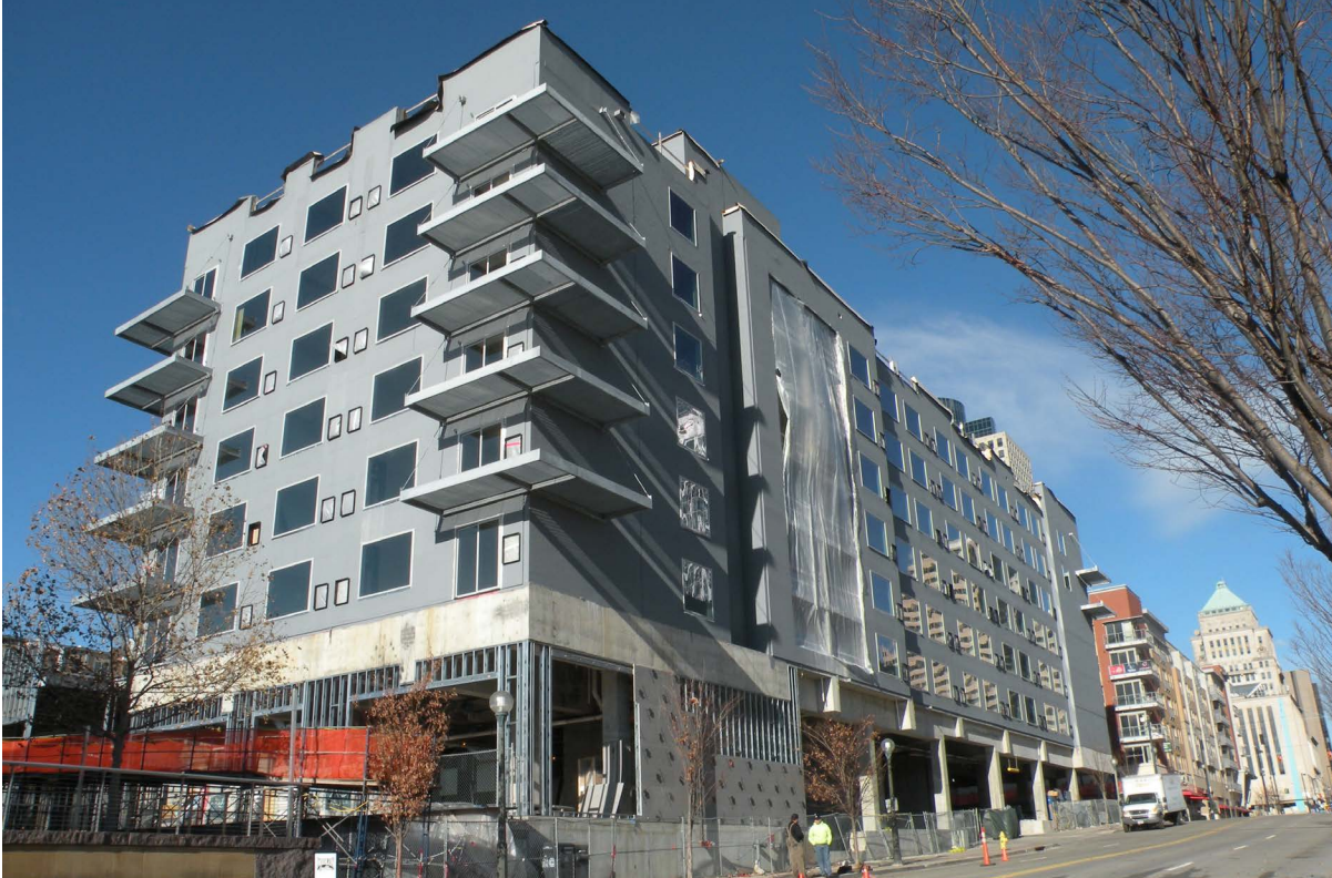
The 171-room AC Hotel construction is expected to be complete in 2017.
