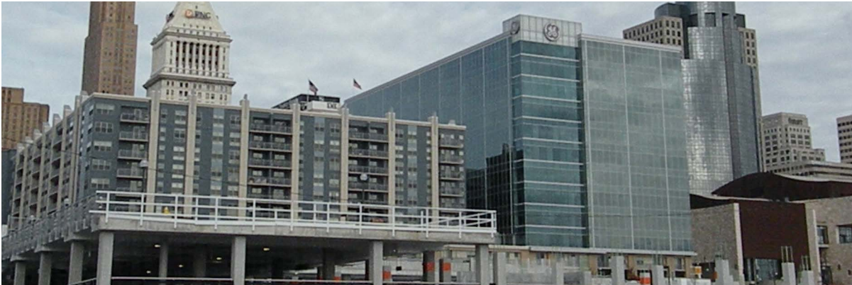
The Radius Apartments and the GE Global Operations Center (part of the Developer's Phase IIA) were completed in 2016. Phase IIIA infrastructure project is in the foreground.
