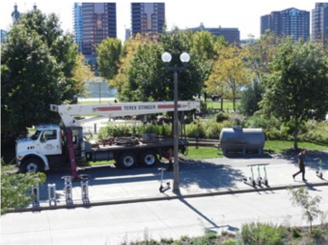
Geothermal well cleaning and pump maintenance.
