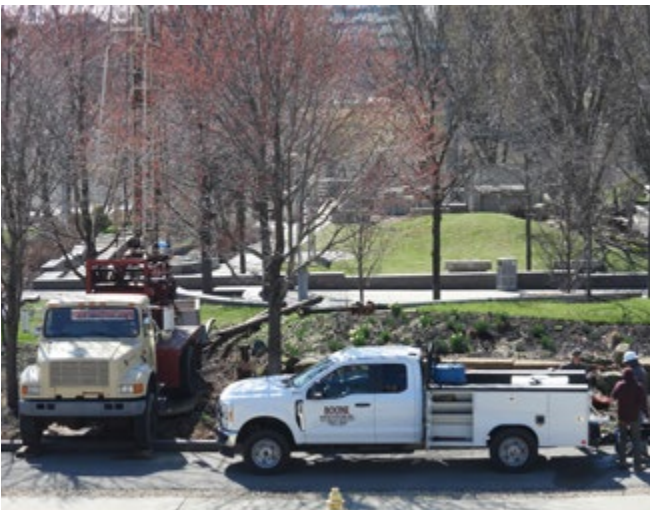
Maintenance work on the geothermal wells beneath Smale Riverfront Park.
