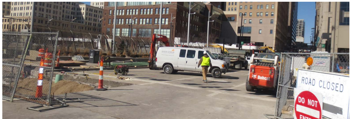
Work on Second Street at Walnut.
