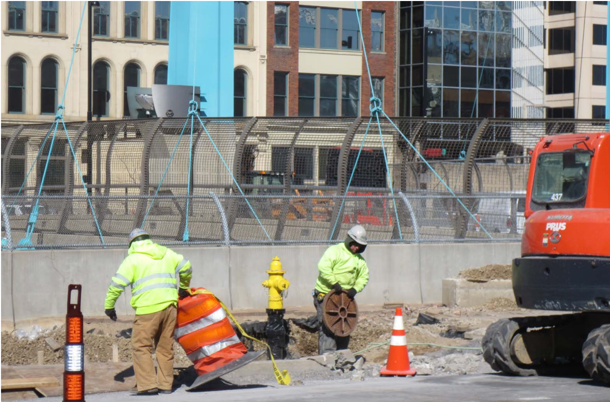
Second Street north sidewalk utility work.
