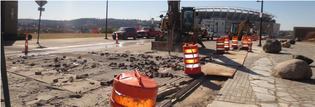
Freedom Way demolition.
