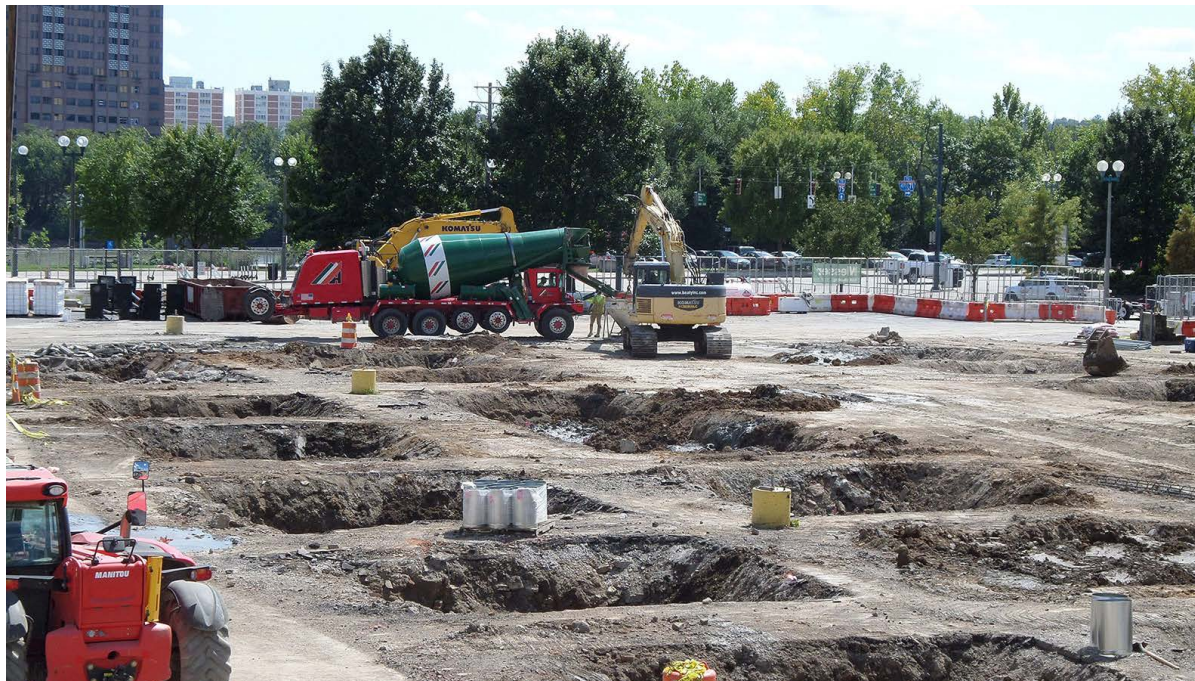
Crews dig production pile pits for Phase IIIB infrastructure in Lot 27.
