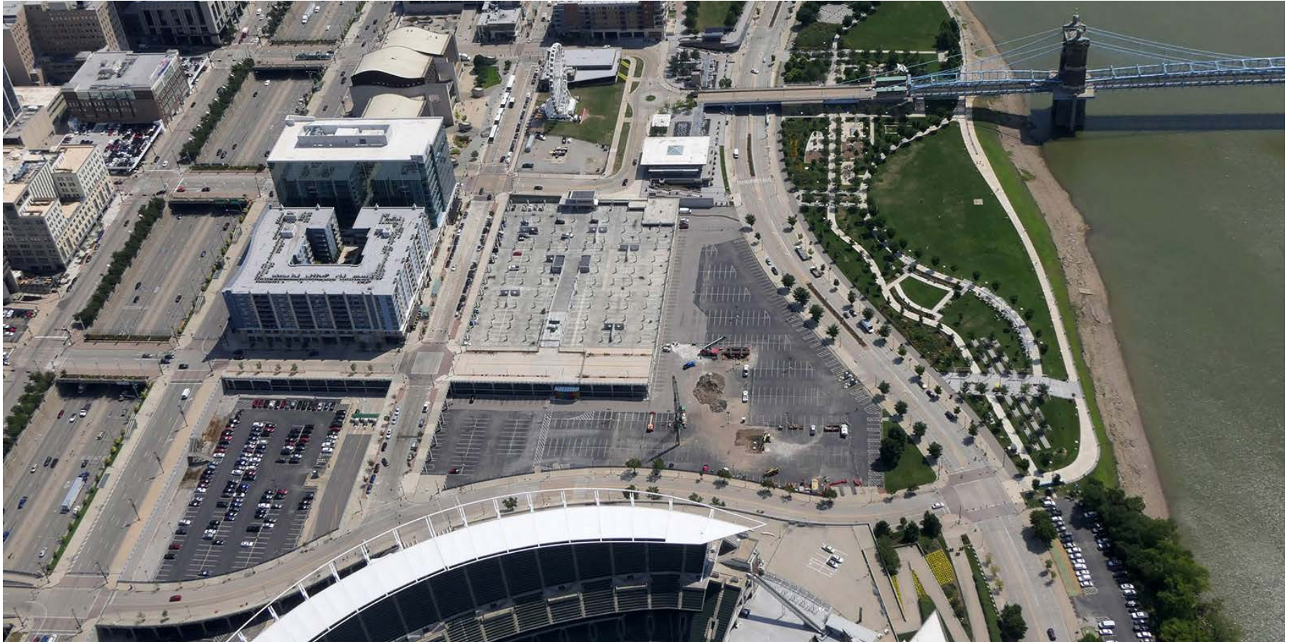
Aerial view of the Phase IIIB work area, viewed from Paul Brown Stadium looking east.
