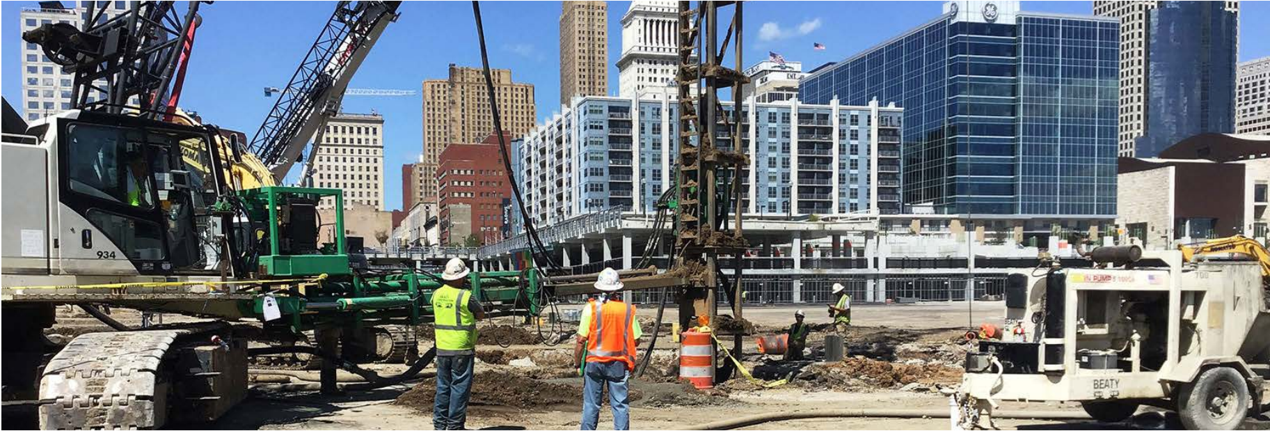
The production pile process gets underway.
