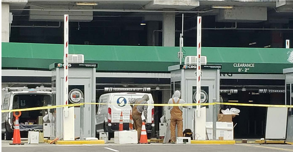
Installation of new enter/exit equipment continued throughout the Central Riverfront Garage.
