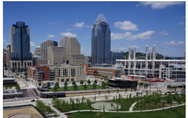
Figure 11. Completed first phase of the mixed-use development viewed from southwest with the ballpark on the right, the buildings on Third Street in the background and the phase 1 park in the foreground (November 2011)
